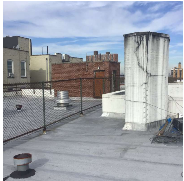
Roof 1 - North View
