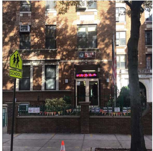
Facade A - Ovington Avenue
