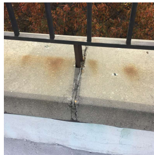
Roof 1 - Facade A
