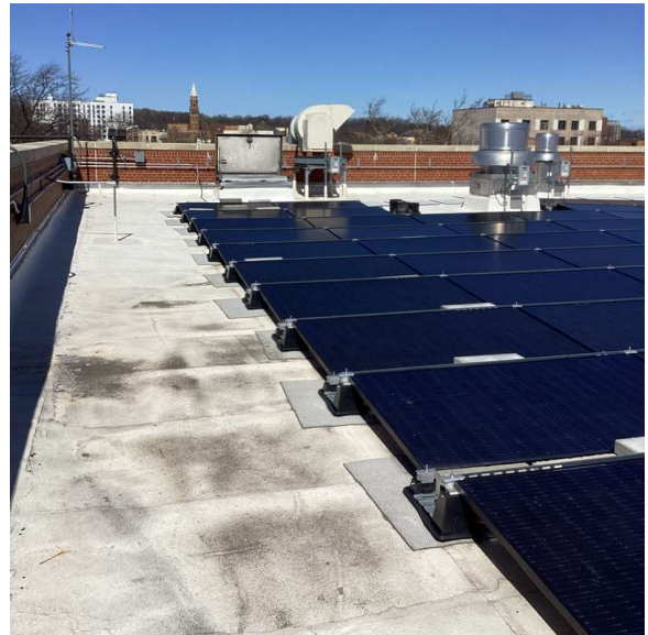
Roof 1 - North View
