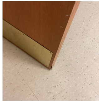
Corridor near Room 209-1
