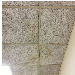
Corridor near Exit 2
