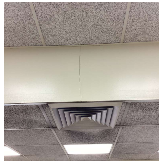
Main Entrance Stair Lobby
