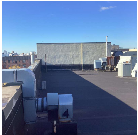
Roof 1 - West View
