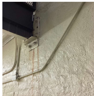
Roof 2 - Stair A/5
