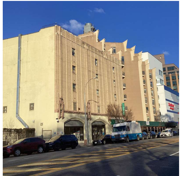
Coney Island Avenue - West View
