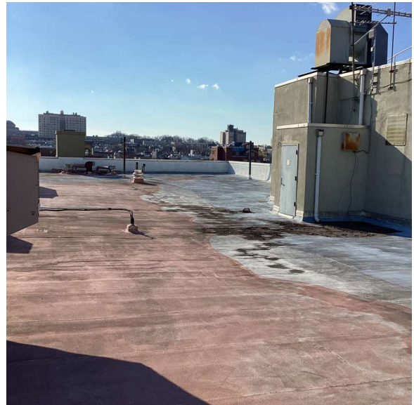
Roof 1 - Southeast View
