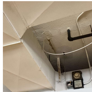
Roof 1 - Room 609 - Shown (Similar: Rooms 617, 619, 619B)
