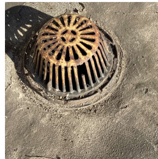
Roof 1 - Near BH2
