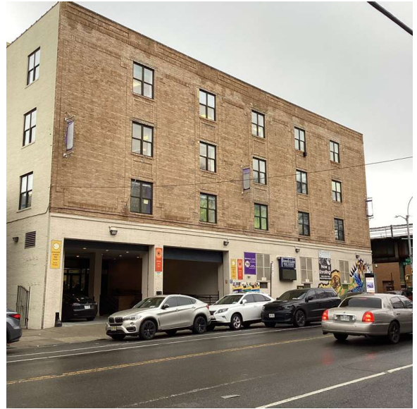
East New York Avenue - South View
