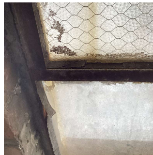
Roof 1 - Elevator Machine Room
