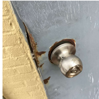
Roof 1 - Elevator Machine Room
