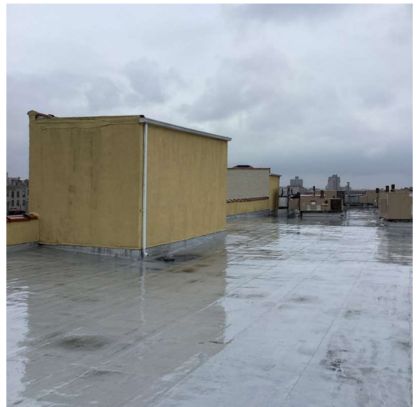
Roof 1 - Northwest View
