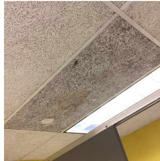
Boys Toilet Room - 4th Floor No violations recorded.
