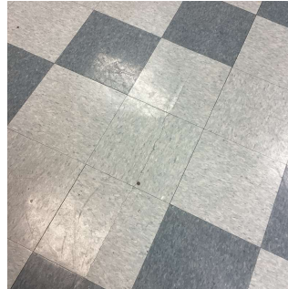
Near Main Entrance
