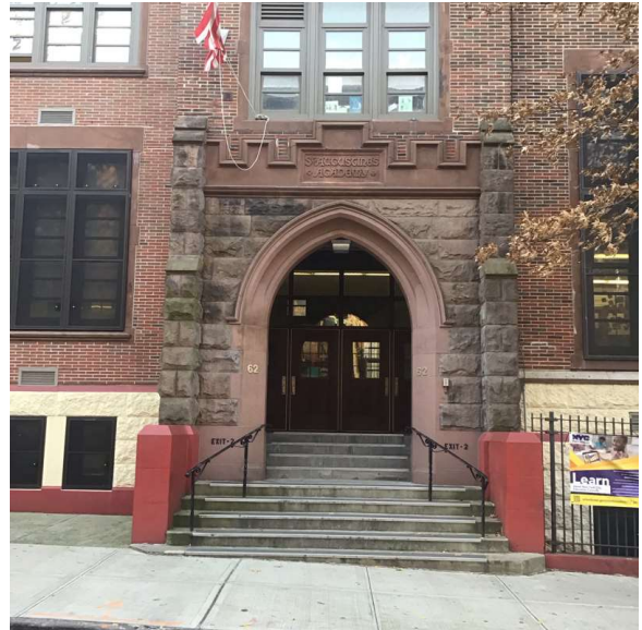
Facade A - Park Place
