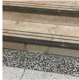
Corridor near Room 312
