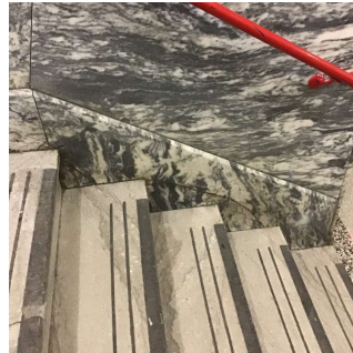
Corridor near Room 304
