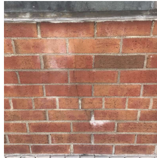
Roof 1 - Facade F
