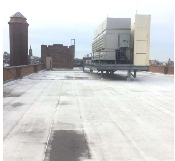
Roof 1 - Southwest View
