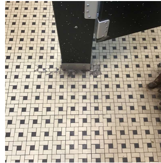
Girls Toilet Room - 4th Floor
