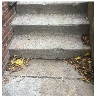
Northeast corner stair in Courtyard
