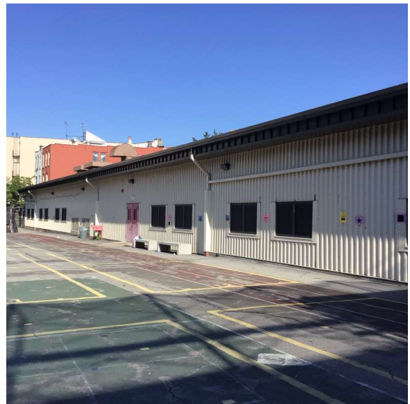
2nd Street - North View
