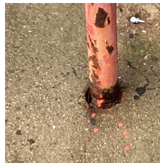
Facade C No violations recorded.
