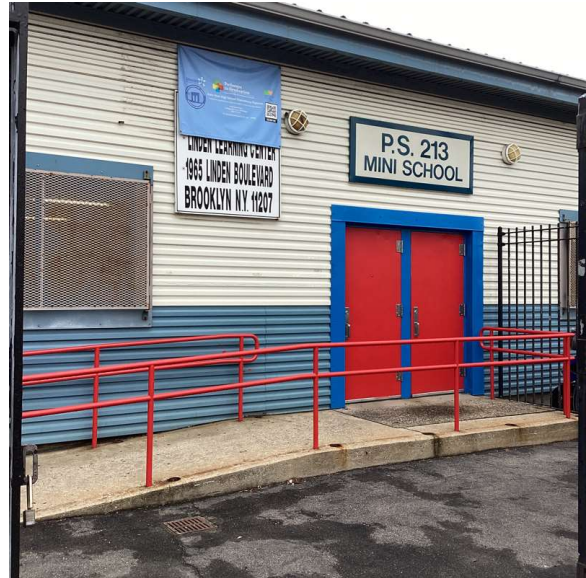
Facade A - Linden Boulevard
