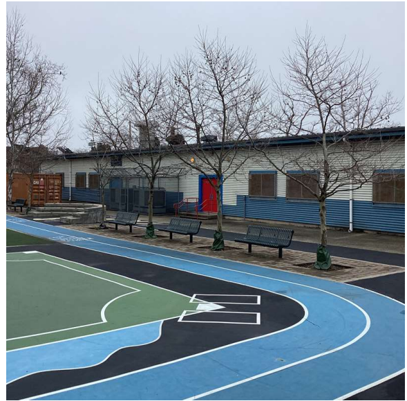
Facade C - Southeast View
