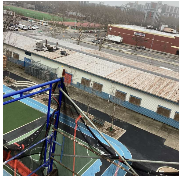
Roof 1 - Southeast View
