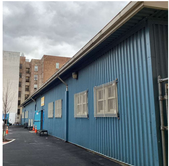
Playground - Southeast View
