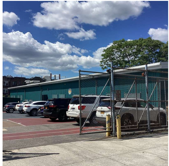
East New York Avenue - Southwest View
