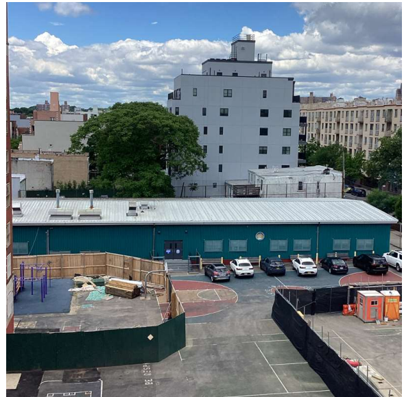
Roof 1 - West View
