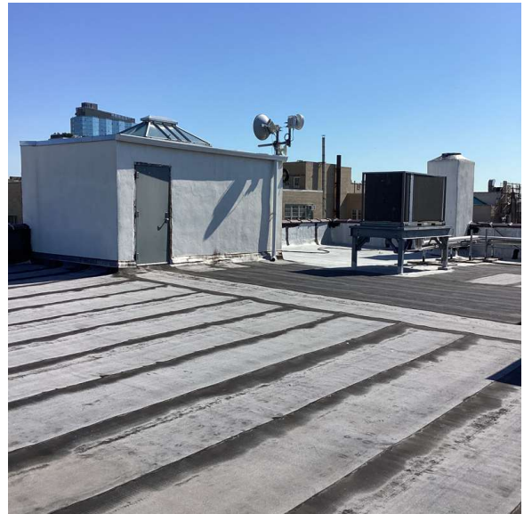
Roof 1 - Northeast View
