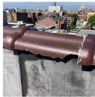
Roof 1 - Facade B No violations recorded.
