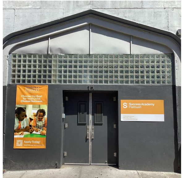
Facade A - Snyder Avenue
