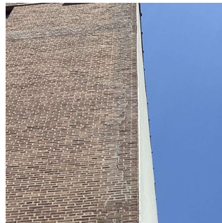
Corner of Facades A and D
