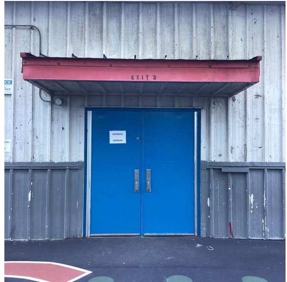
Facade A - Schoolyard
