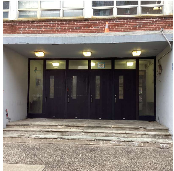
Facade A - Crown Street
