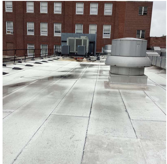
Roof 1 - East View
