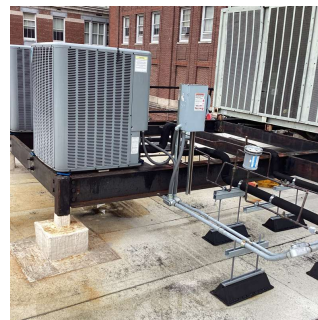
Roof 1 No violations recorded.
