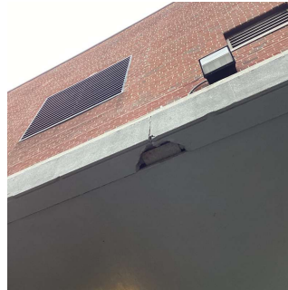
Facade A - Main Entrance No violations recorded.
