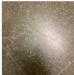
Right side stage vestibule No violations recorded.
