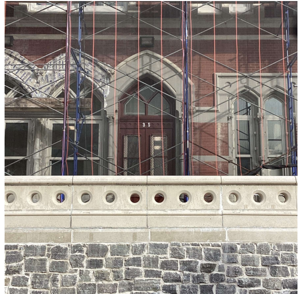
Facade A - Snyder Avenue
