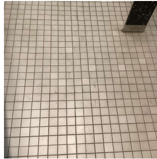
Women Toilet Room - 1st Floor
