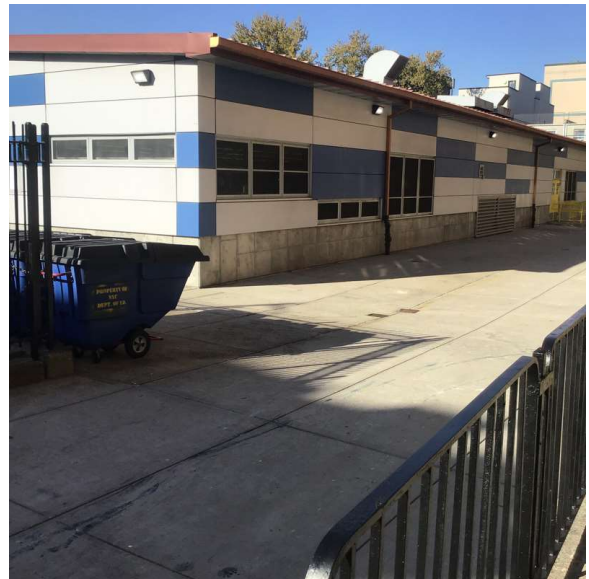
Kosciuszko Street - West View
