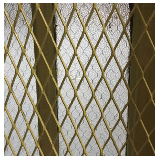
Facade B - Stairwell A/3 and A/1
