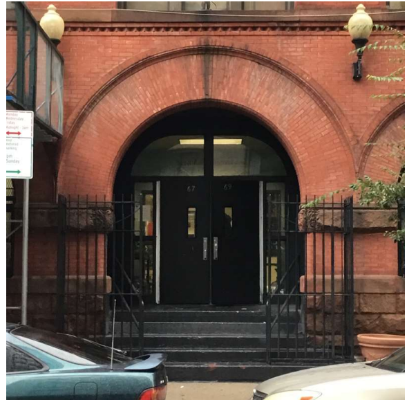
Facade A - Schermerhorn Street
