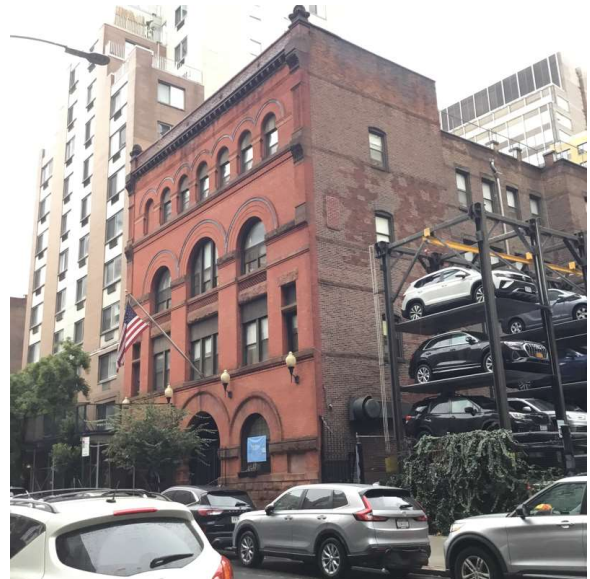
Schermerhorn Street - North View
