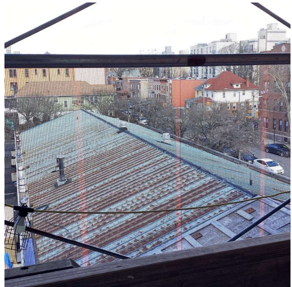
Roof 1 - North View
