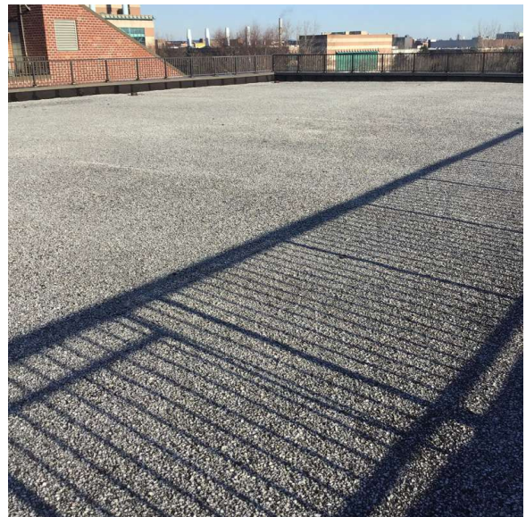
Roof 1 - North View
