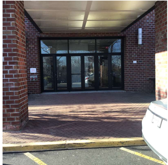
Facade A - Van Siclen Avenue
