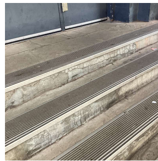
Facade A No violations recorded.
