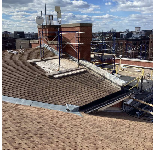
Roof 1 - Southwest View
