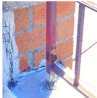
Roof 1 No violations recorded.
