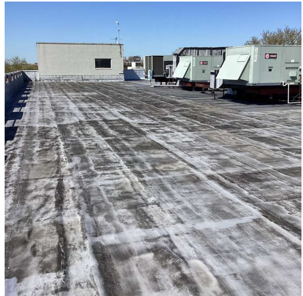
Roof 1 - West View
