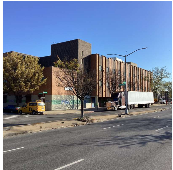
Corner of Linden Boulevard and Bradford Street - Northeast View
