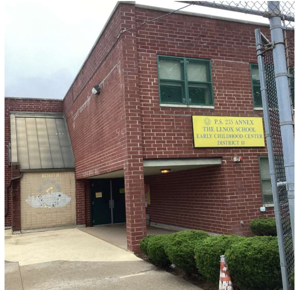
Facade A - East 58th Street
