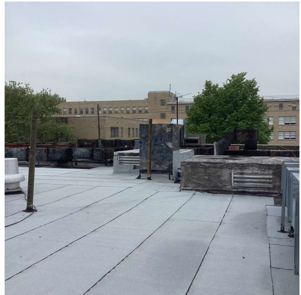
Roof 1 - West view
