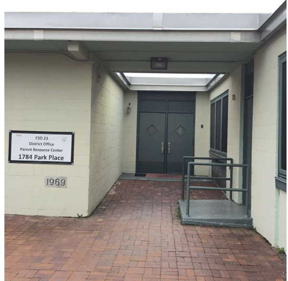
Facade A - Park Place
