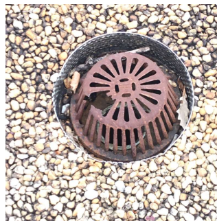
Roof 1 No violations recorded.
