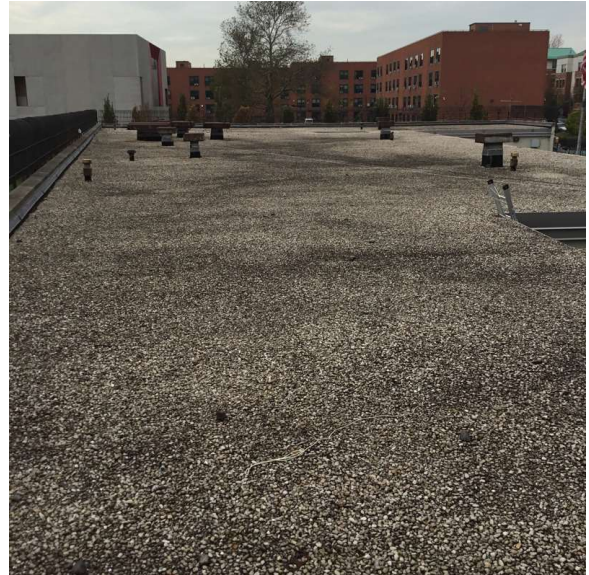
Roof 1 - West View
