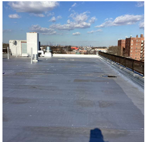
Roof 1 - North View
