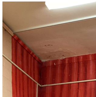
Roof 2 - Multipurpose Room (shown), Multipurpose Room Office No violations recorded.
