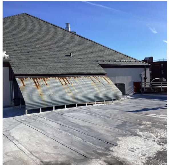
Roof 1 - Southwest View
