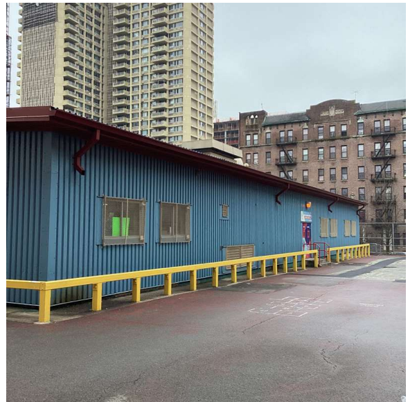
Facade A - Southeast View
