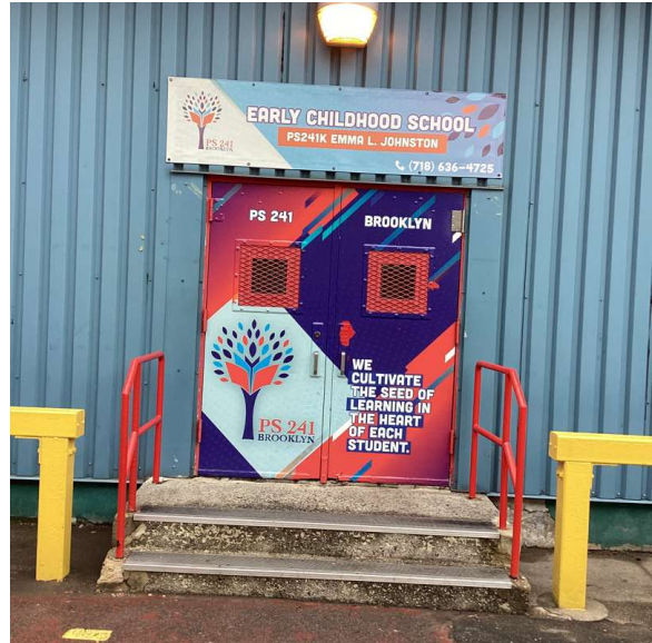
Facade A - East View
