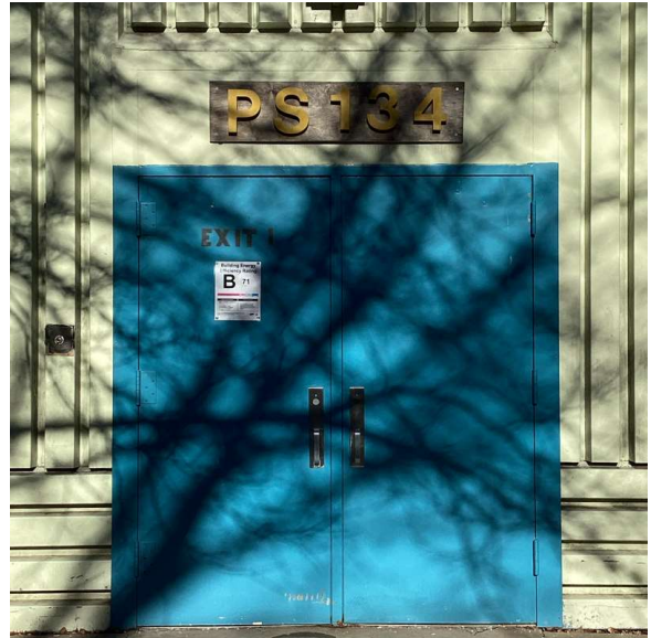
Facade A - Webster Avenue
