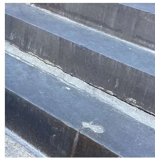
Facade D - Exit 8
