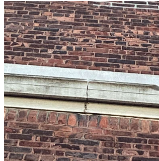
Facade D - Near Exit 9
