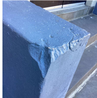
Facade D - Exit 8 No violations recorded.
