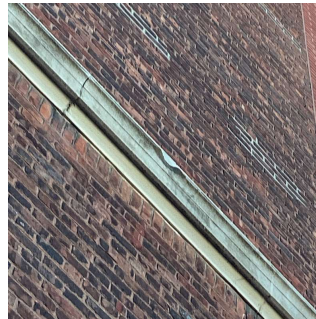
Facade D - Near Exit 9
