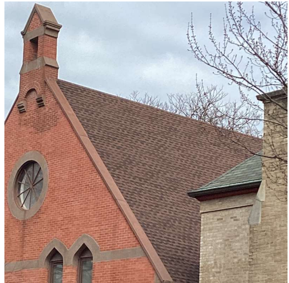
Roof 1 - Northeast View
