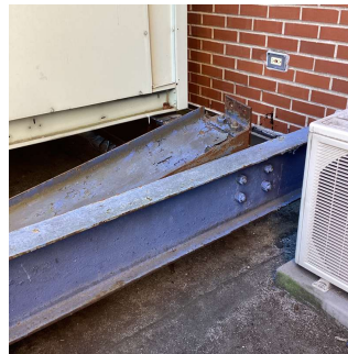
Roof 5 No violations recorded.
