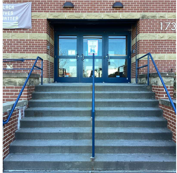
Facade A - Conover Street
