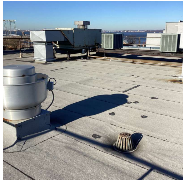
Roof 1 - West View
