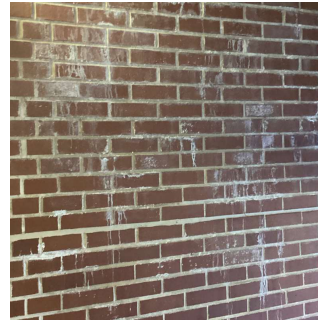
Facade B - Stairwell A/3 (Facade B - Stairwell A/2 similar)
