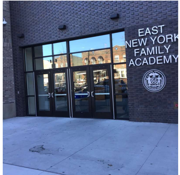
Facade A - Van Siclen Avenue
