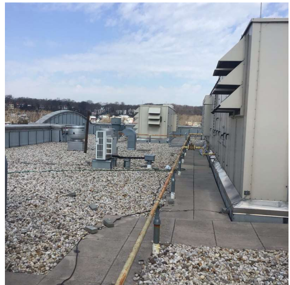
Roof 1 - Northwest View
