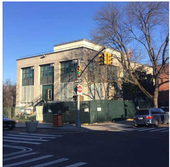
Corner of Park Place and Underhill Avenue - Northeast View
