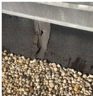
Roof 1 - Facade E
