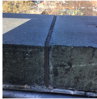
Roof 1 - Facade C
