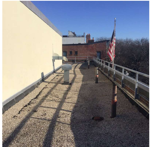
Roof 1 - East View
