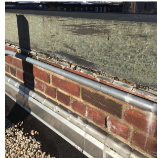
Roof 1 - Facade C
