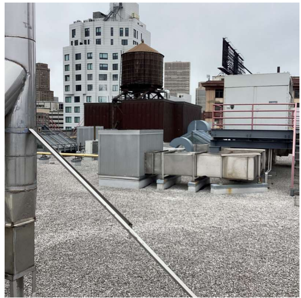
Roof 1 - Southwest View
