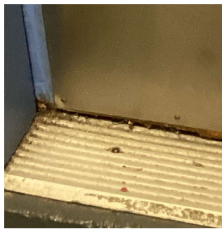
Facade B - Exit 3 No violations recorded.
