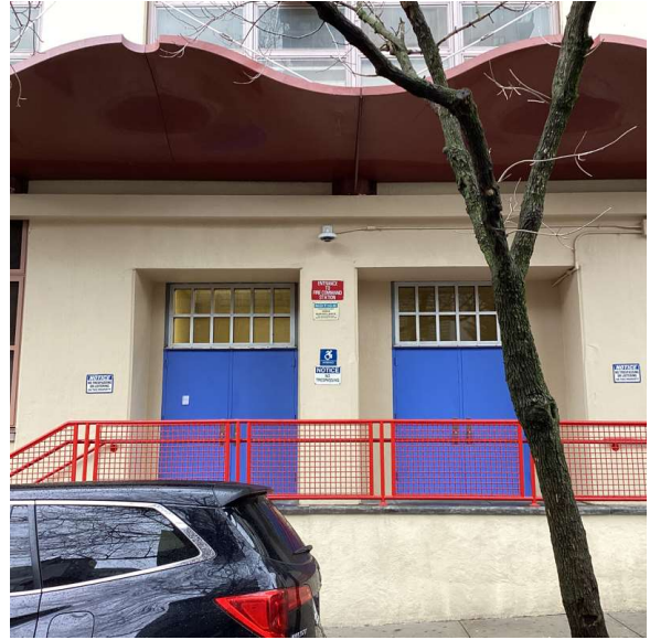
Facade A - Concord Street
