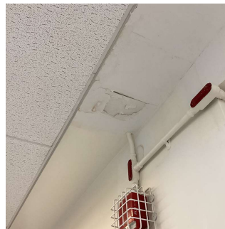
Roof 1 - Corridor near Room 814 shown, Roof 1 - Rooms 812, 819, Corridor near Rooms 804, 806 similar
