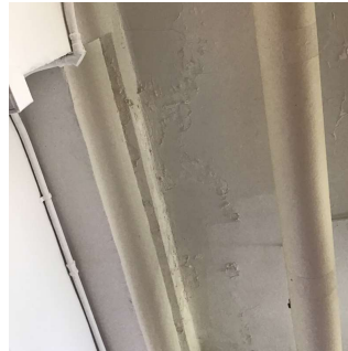
Corridor near Room 411
