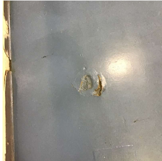
Near Windows No violations recorded.
