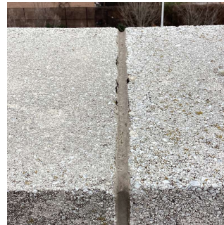
Roof 1 - Facade J
