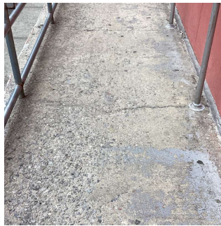
Facade J - HC Ramp
