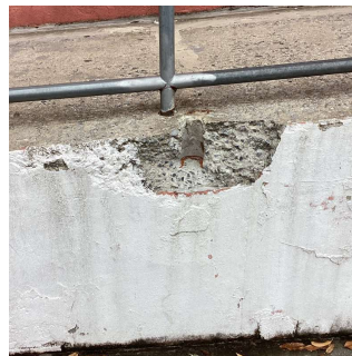
Facade J - HC Ramp
