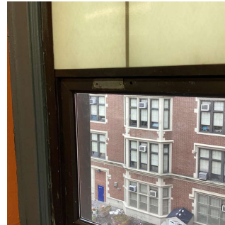
Facade L - Corridor near Room 415
