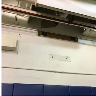
Near Girls Locker Room No violations recorded.
