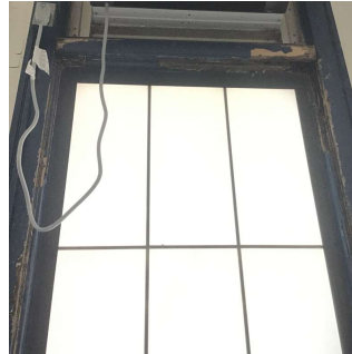
Facade L -Room 314
