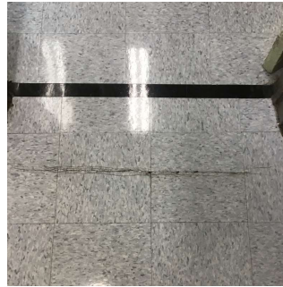
Corridor near Room 607
