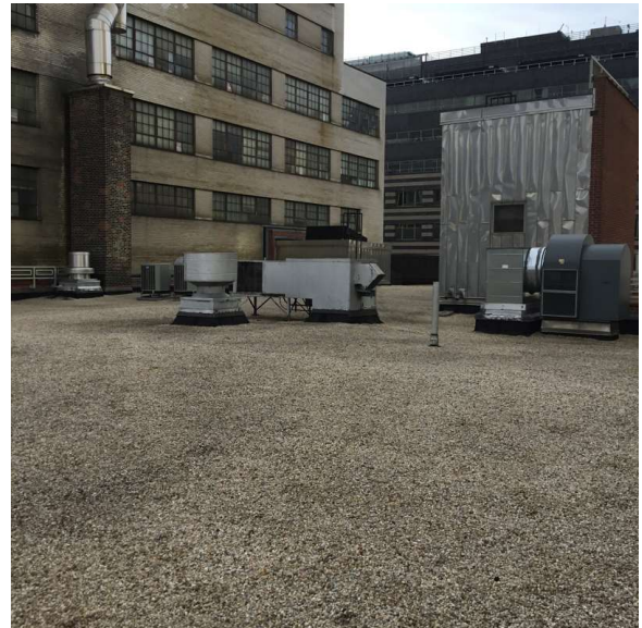
Roof 1 - Southeast View
