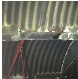
Basement Storage Room (Parking Garage, Oil Tank Room similar)
