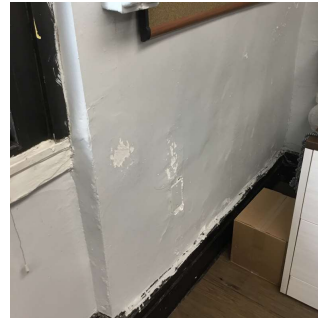
Facade A - Room 501B (Facade A - Room 401B similar)
