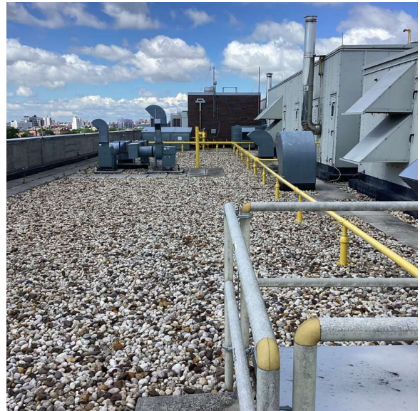
Roof 1 - Southwest View
