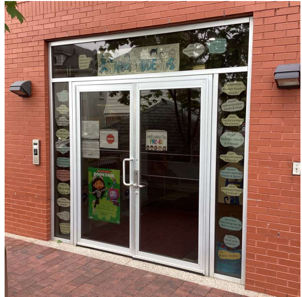
Facade A - East View
