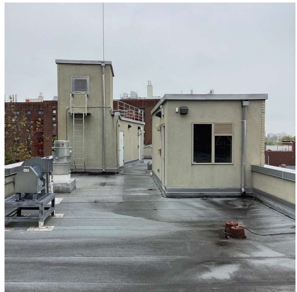
Roof 1 - Southeast View
