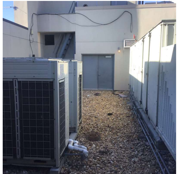
Roof 1 - West View
