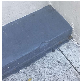
Facade A - North End No violations recorded.
