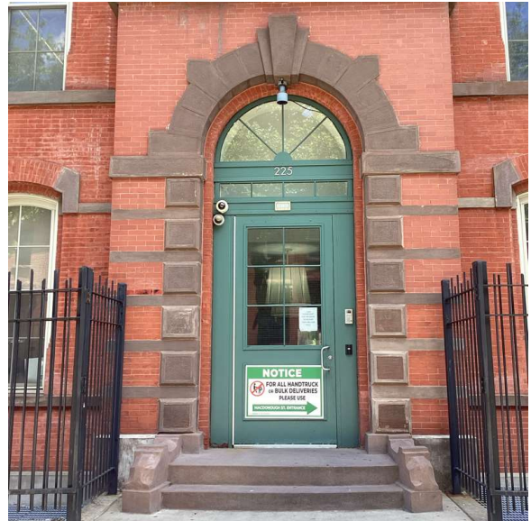
Facade A - Patchen Avenue
