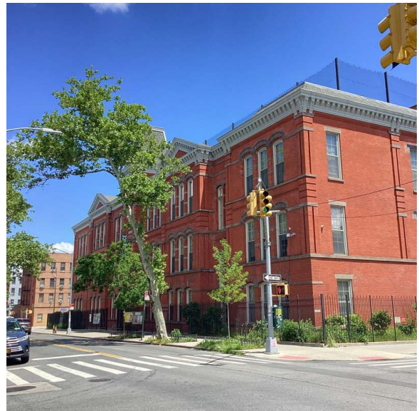
Corner of MacDonough Street and Patchen Avenue - Northeast View
