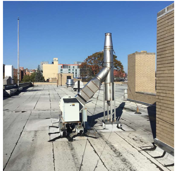
Roof 1 - Northwest View
