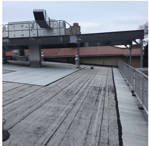
Roof 1 - Southeast View
