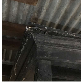
Facade A - Exit 5
