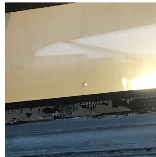
Facade C - Exit 3
