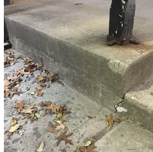
Facade A - Exit 5
