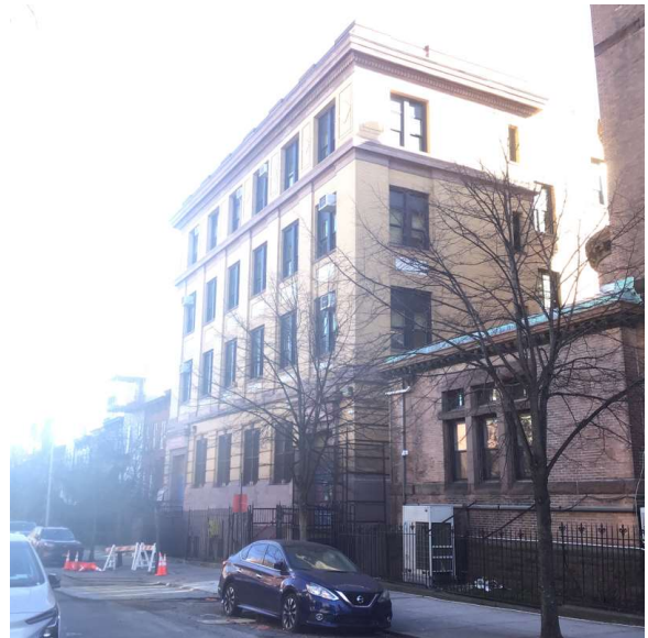
Corner of Hooper Street and Marcy Avenue - Northeast View
