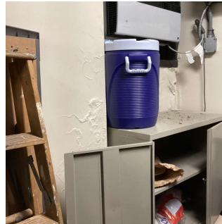
Facade B - Room 105 (shown), Multipurpose Room, Stair B/3 No violations recorded.
