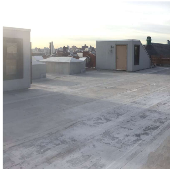
Roof 1 - Southeast View
