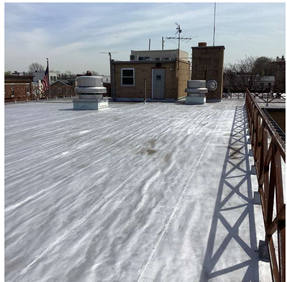
Roof 1 - Southeast View
