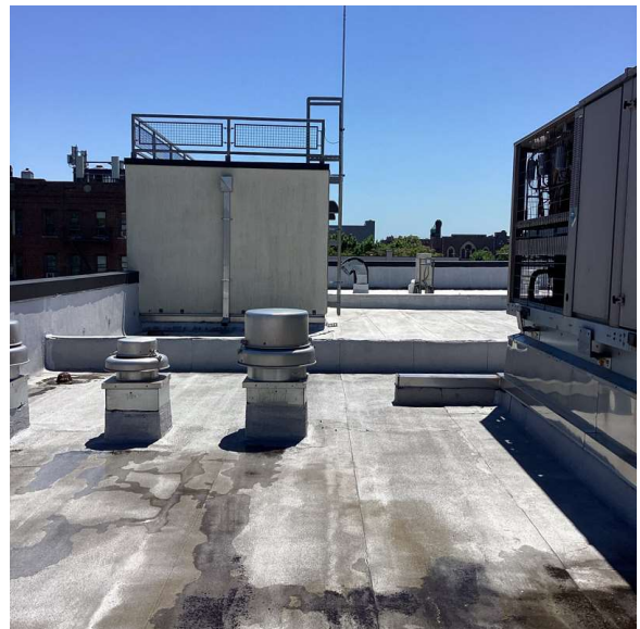
Roof 1 - Northeast View
