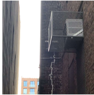
Chimney - Facade M
