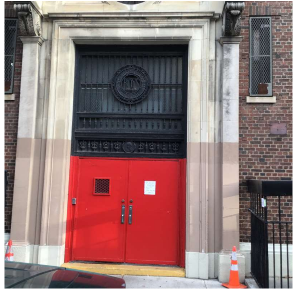
Facade A - 8th Street
