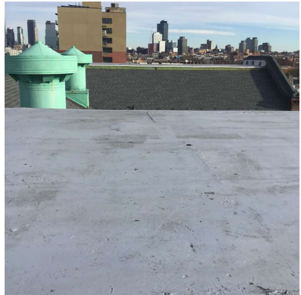
Roof 1 - Northeast View
