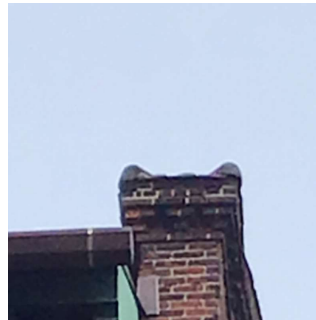
Facade H No violations recorded.
