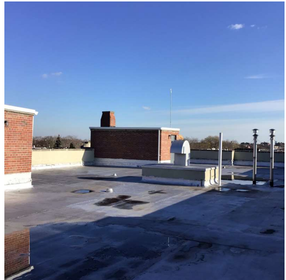
Roof 1 - West View
