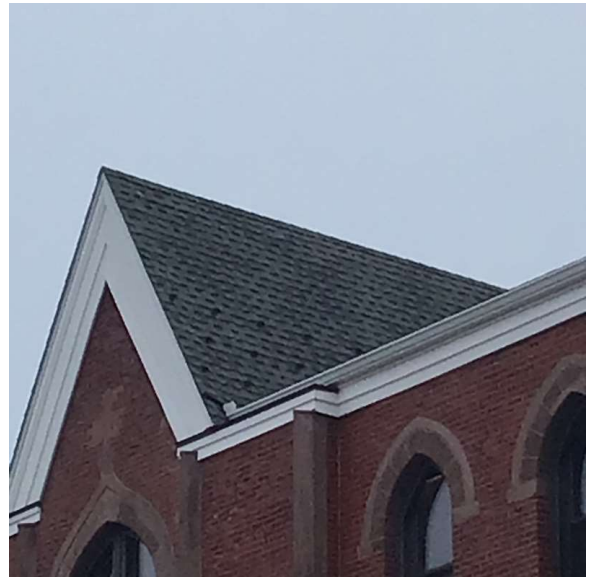
Roof 1 - North View
