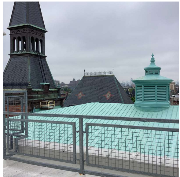
Roof 2 - Northwest View
