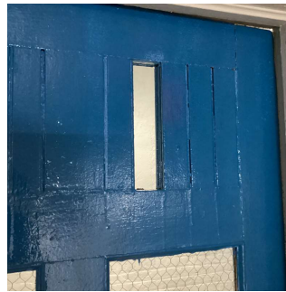
Basement Exit 2 Vestibule
