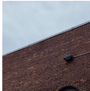
Roof 2 - Facade D No violations recorded.
