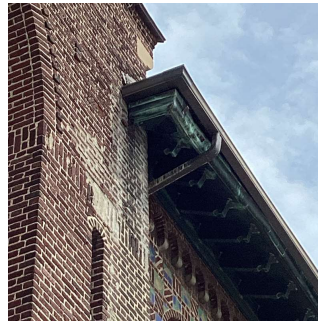
Roof 1 - Facade A
