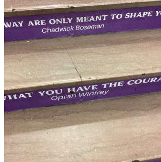
Left Side Lobby Stair
