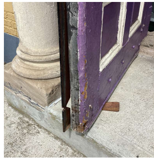
Facade A - Main Entrance No violations recorded.
