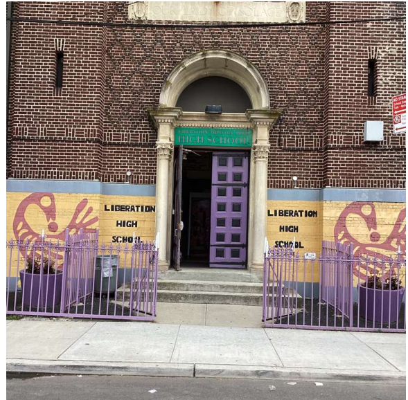
Facade A - West 19th Street
