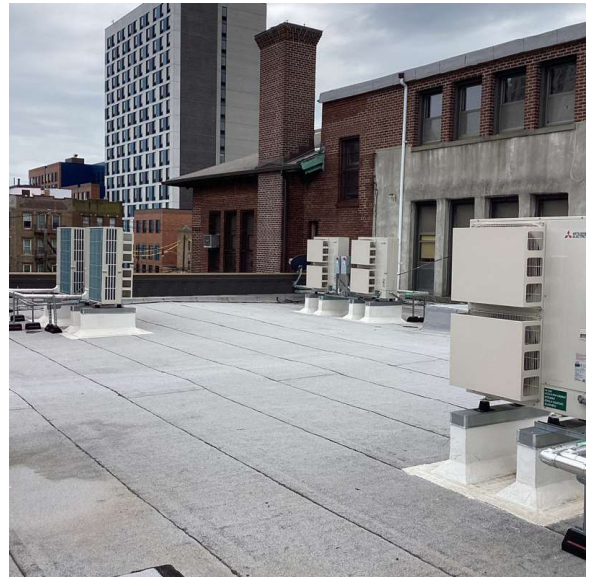
Roof 2 - Southwest View
