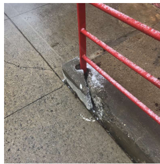
Facade D - Service Ramp No violations recorded.
