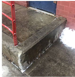
Facade D - Service Ramp
