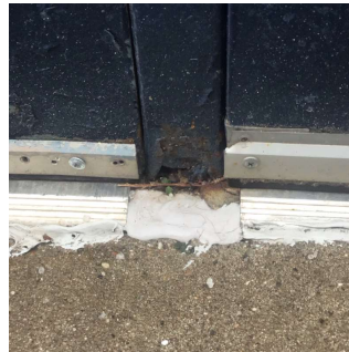
Facade C - Exit 1
