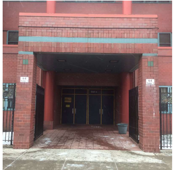
Facade A - Avenue X
